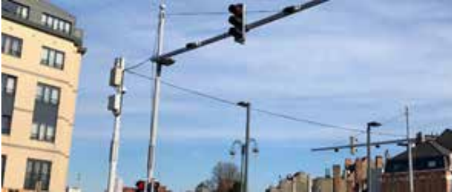
Source: ANPR cameras mounted on the pole of a traffic light in Koekelberg
